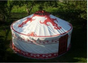
The structure of a yurt consists of a wooden lace forming a wall, about 40 supports connected to the wheel at the top, two pillars supporting the wheel and doors of solid wood. Such a structure is covered by a <u>canvas cover</u>. If the yurt will be used only during spring and autumn, you do not need to buy mount insulation. The whole construction is **extremely robust and resistant to even very strong winds.**
