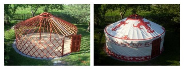
The structure of a yurt consists of a wooden lace forming a wall, about 40 supports connected to the wheel at the top, two pillars supporting the wheel and doors of solid wood. Such a structure is covered by a <u>canvas cover</u>. If the yurt will be used only during spring and autumn, you do not need to buy mount insulation. The whole construction is **extremely robust and resistant to even very strong winds.**
