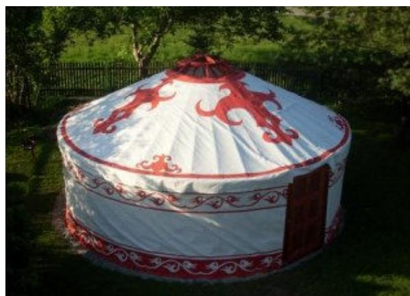
The structure of a yurt consists of a wooden lace forming a wall, about 40 supports connected to the wheel at the top, two pillars supporting the wheel and doors of solid wood. Such a structure is covered by a canvas cover. If the yurt will be used only during spring and autumn, you do not need to buy mount insulation. The whole construction is **extremely robust and resistant to even very strong winds**.
