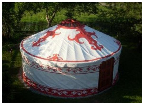
The structure of a yurt consists of a wooden lace forming a wall, about 40 supports connected to the wheel at the top, two pillars supporting the wheel and doors of solid wood. Such a structure is covered by a canvas cover. If the yurt will be used only during spring and autumn, you do not need to buy mount insulation. The whole construction is **extremely robust and resistant to even very strong winds**.
